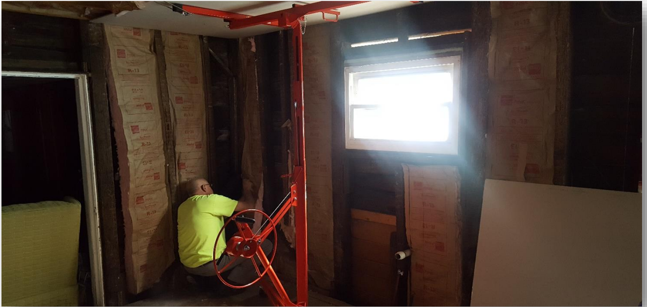
John Holt insulating wall with drywall lift supporting sheet on ceiling
