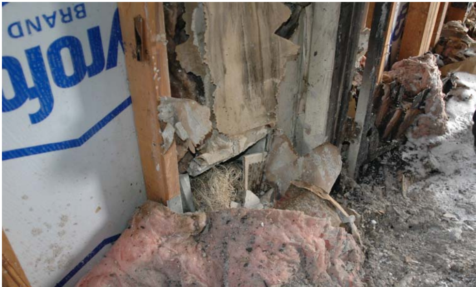
Excelsior fire loading in vents between wall studs.
