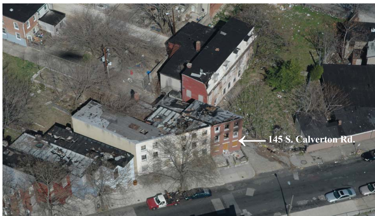
Picture shows exposures to B and D sides of structure.
