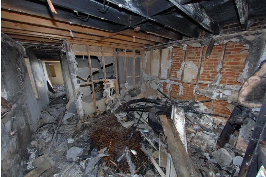
Debris in rear room prior to removal.
