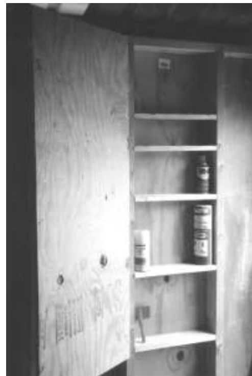
Lockable shelf constructed between wall studs in the toolshed
