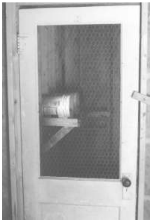
"Screen door" made by cutting out
