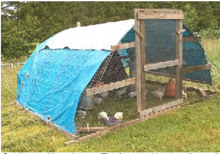
Cattle-panel hoophouse. The front and back walls are framed with 1x4 lumber and covered with chicken wire. The door is a hatch that lifts out. Photo: Robert Plamondon
