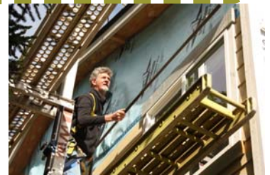
Doug Pugsley installing siding
